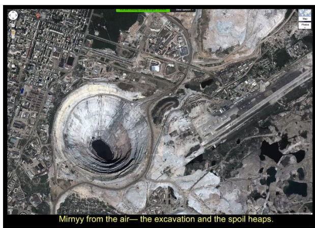
Mirny from the air – excavation & spoil heaps
