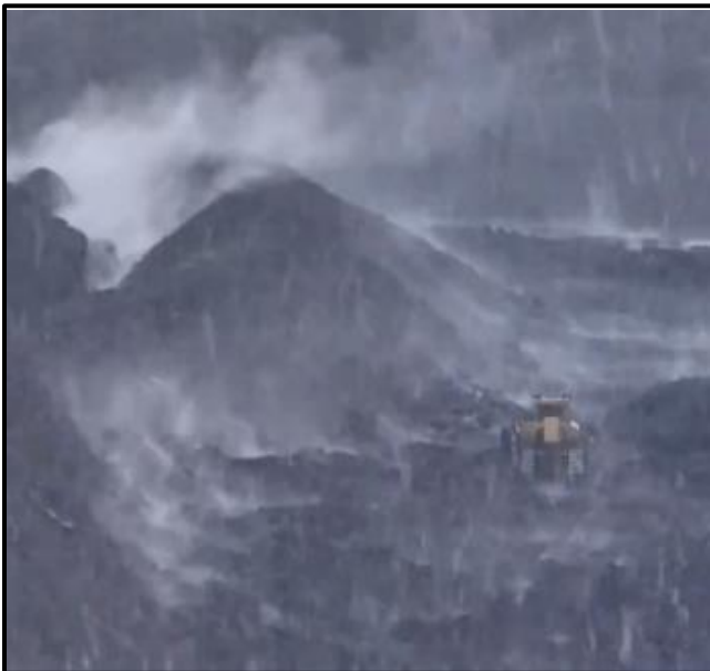
Lone bulldozer at work during snowstorm and fumes of sulfur dioxide, constructing walls of basalt to divert new lava flows. Isak’s video on March 21, 2024, Isak’s drone.
